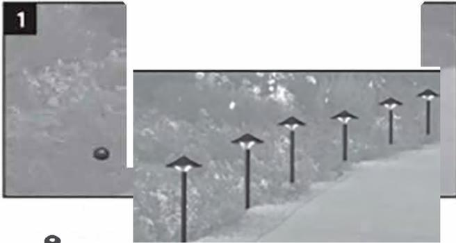
1. Locate placement of lights and lead wiring. If you choose bury wire under concrete or other permanent structures, plan accordingly.
