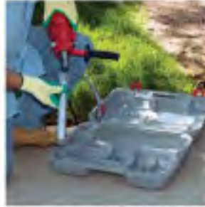
Attach Diamond Core Bit
