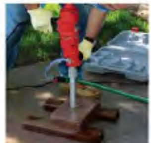
add pressure and drill through paver.
