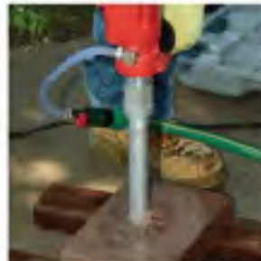
As drill bit gets started, straighten to 90°
